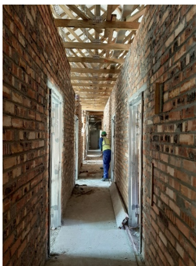
Reconstruction work in progress.
