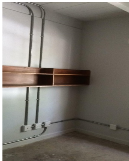
New electrical and data installation in a bedroom.
