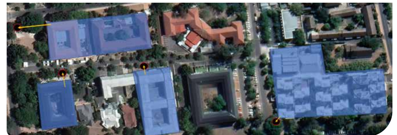
Aerial view of the Stellenbosch University campus showing residences with manholes. Image: Edward Archer
