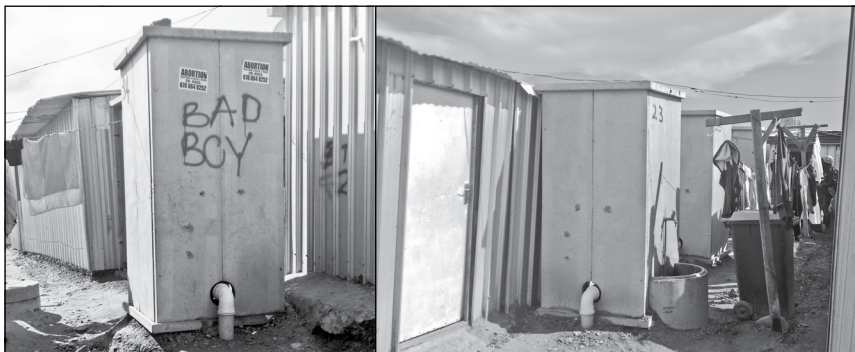
Image 1: Mshini Wam – 2013: Location of toilet structures in a re-blocked section
