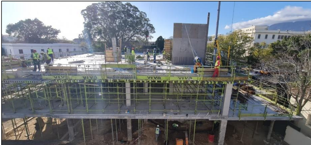
Second floor of Victoria hub being completed
