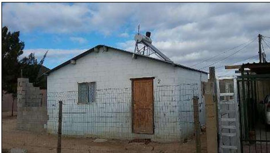
**Figure 25 Example of a typical subsidy house in Klapmuts with no guttering**
