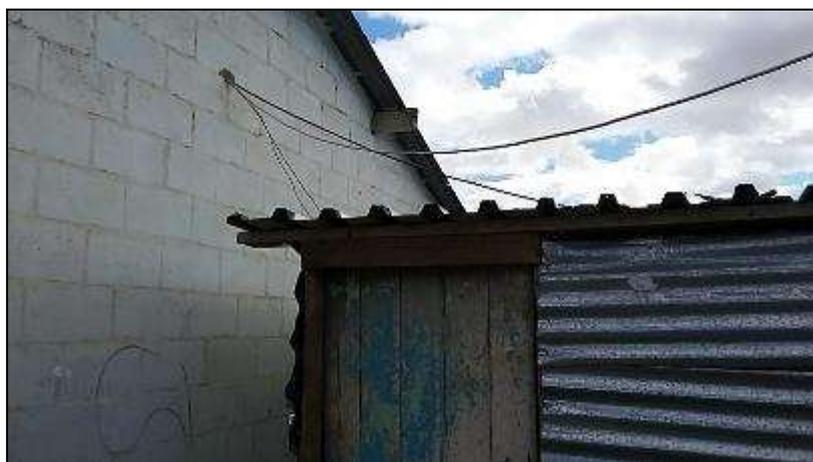
**Figure 19 A typical electricity connection from main house to backyard dwelling**
