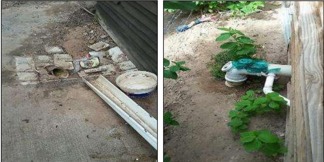
**Figure 18 Examples of ponding and rudimentary drainage/sewage system in backyards**
