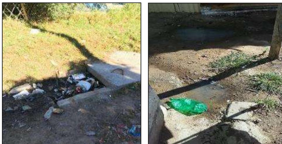
**Figure 17 Typical examples of a blocked stormwater drain and backyard ponding**
