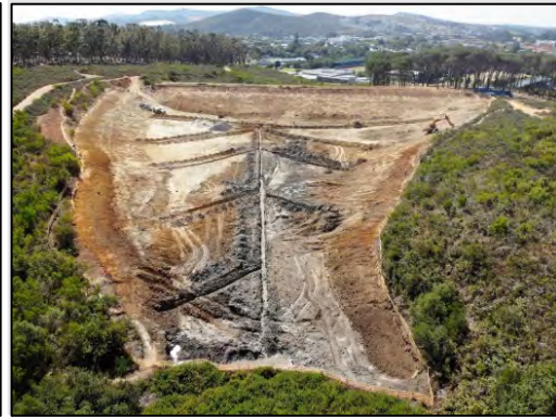
Figure 59: Installation of sub-surface drainage
