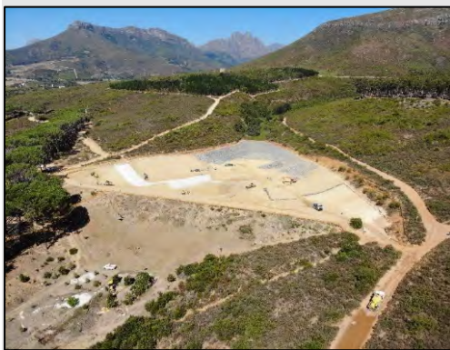
Figure 60: During installation of GC liner
