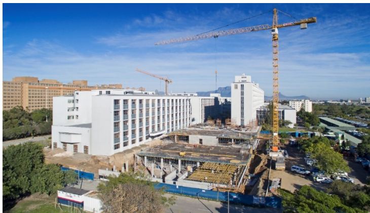
Figure 14: Construction of the new Biomedical Research Institute on Tygerberg campus is progressing well. This photograph was taken on 20 June 2019.
