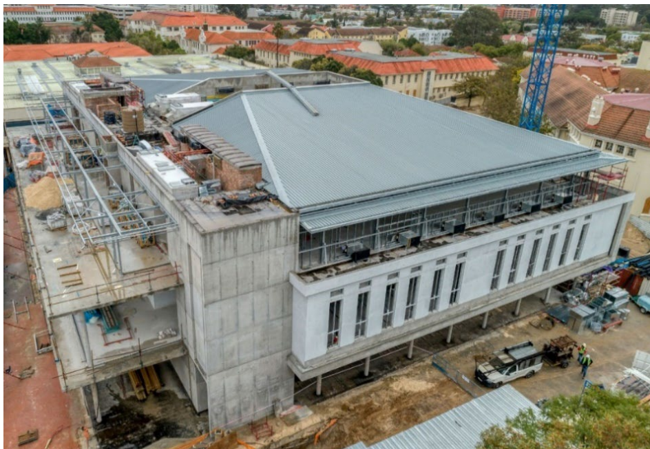
Figure 15: Aerial view of progress on the new Jan Mouton Learning Centre next to the Neelsie.
