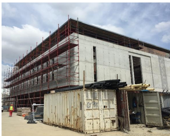
Figure 20: North-eastern corner of the new building
