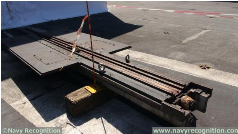
Elements of one of the two aircraft catapults under maintenance.
