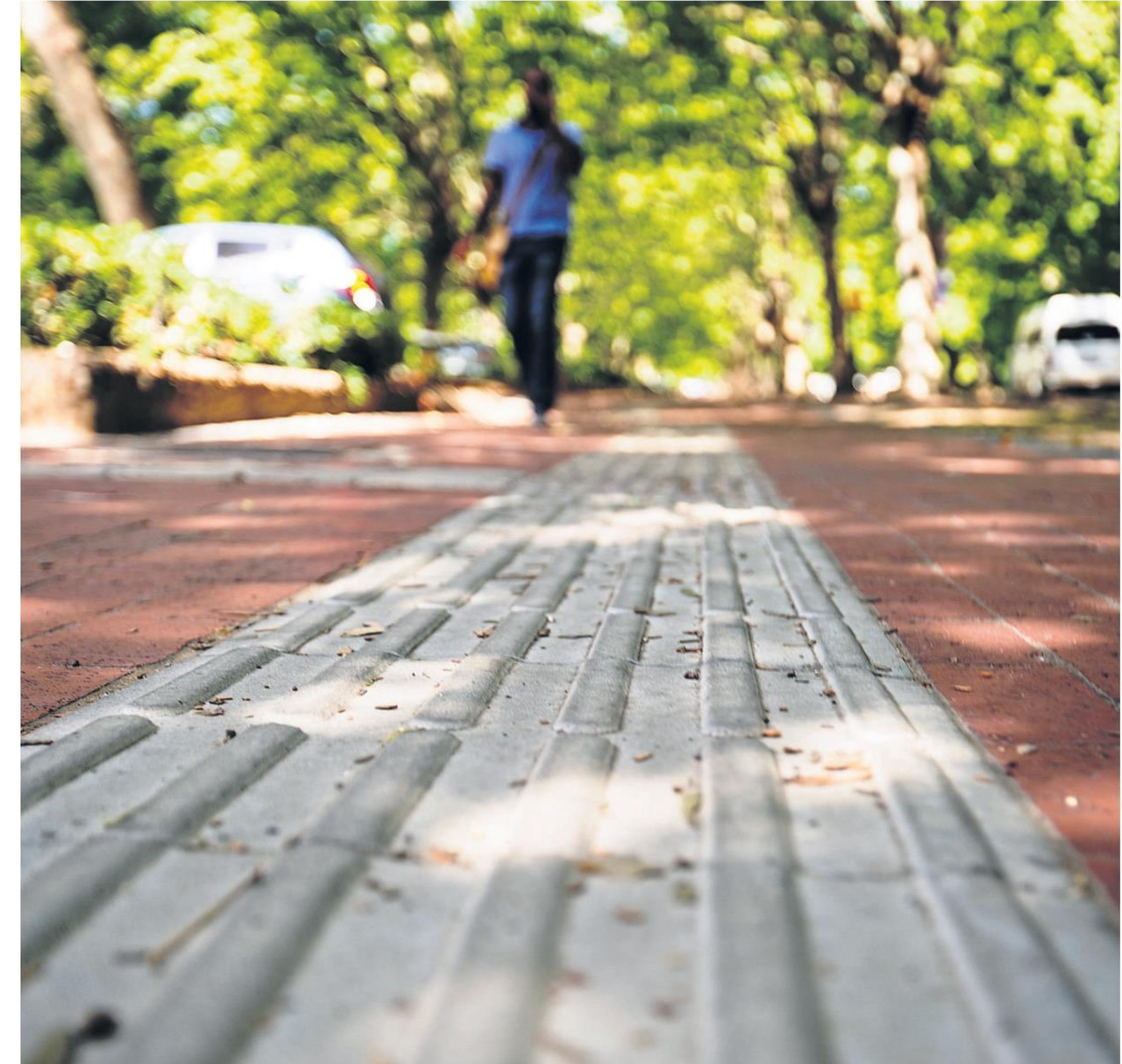
Tactile paving along Victoria Street helps blind students in particular to find their way along busy sidewalks and corners. Tactile paving aids direction and knowing where to cross streets.
