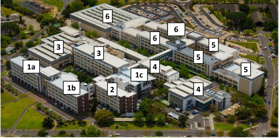
Figure 1.1: The building complex of the Faculty of Engineering (the numbers are used in the descriptions below).
