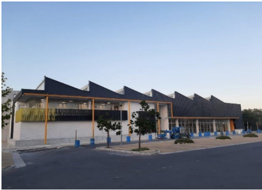
The exterior of the Pavement Laboratory as in March 2020.
