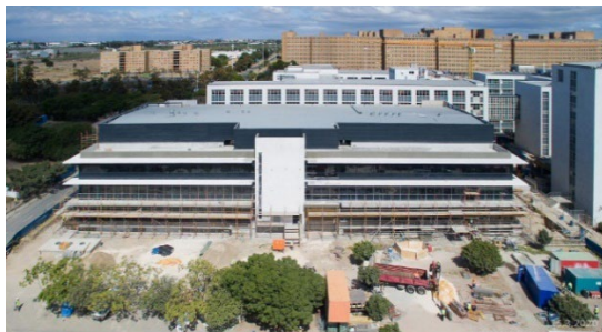
North-facing view of new BMRI building, 24 March 2020.
