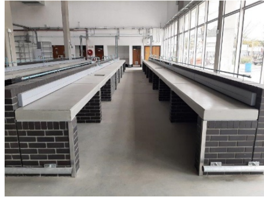
Inside the new building.
