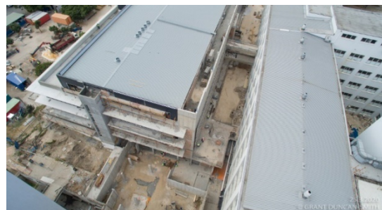
Western view of the new BMRI, showing bridges between the old and new buildings.
