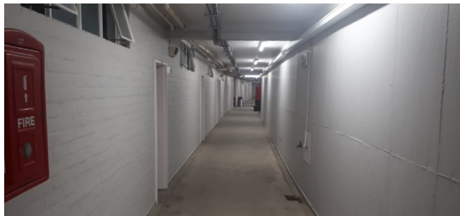
Upgraded pavilion passage and tunnel walkway at the Danie Craven Stadium.
