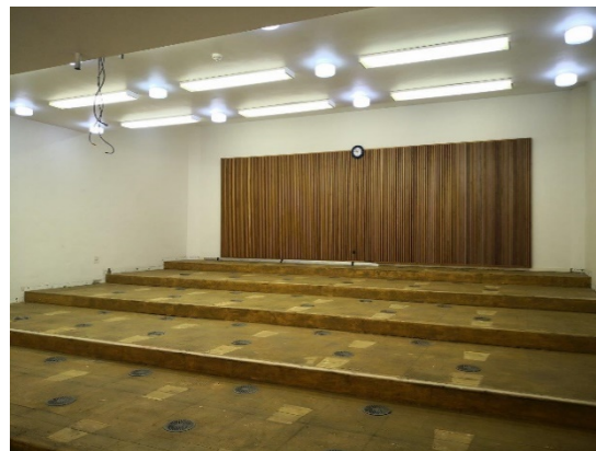
Figuur 71: Lesinglokaal 1027 gedurende sloping.
