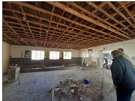
Figure 68: Demolition & removal of floor in kitchen. Figure 69: Removal of old ceilings in servery area.
