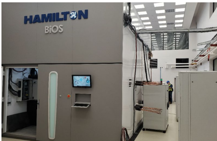
Installation of the Hamilton BiOS at the end of September.
