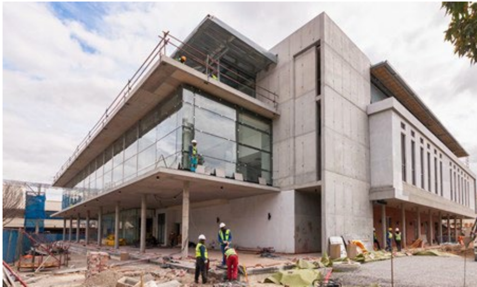
The Jan Mouton Learning Centre is nearing completion.
