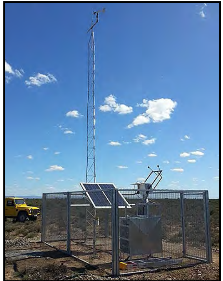
Typical solar radiometric measurement station installed in the Karoo.
